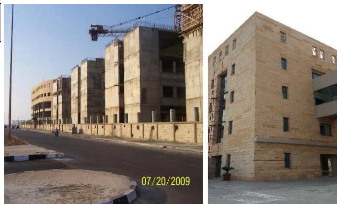
Figure 4: BAU campus under construction and stone cladding.
