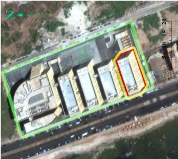
Figure 1: Architectural Faculty Building in BAU Tripoli Campus.
