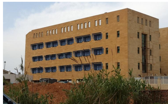
Figure 5: External shading devices proposed for south facade
